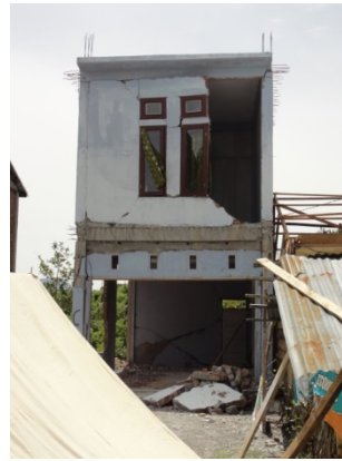
(b) Out-of-plane failure of wall
