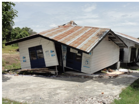
(b) Damage due to spandrel wall collapse
