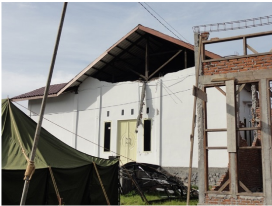
(c) Gable wall failure
