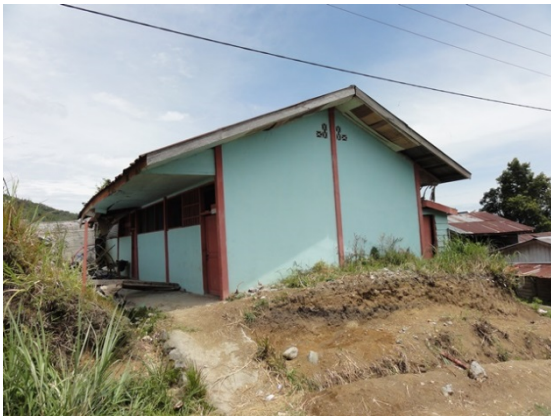
(a) Confined masonry
