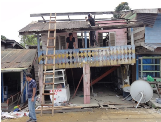
(a) Damage due to ground settlement
