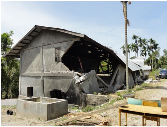
(a) Complete collapse
