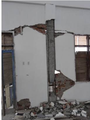
(a) Severely damaged column
