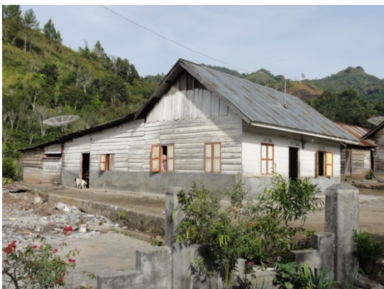
(c) Timber with masonry spandrel walls
