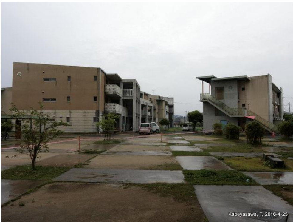
宇土市営団地（周辺地盤の噴砂） Trace of sand boiling at neighborhood ground
