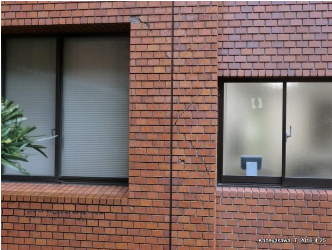
研究棟（短柱のせん断破壊） Shear failure of short column in the new building
