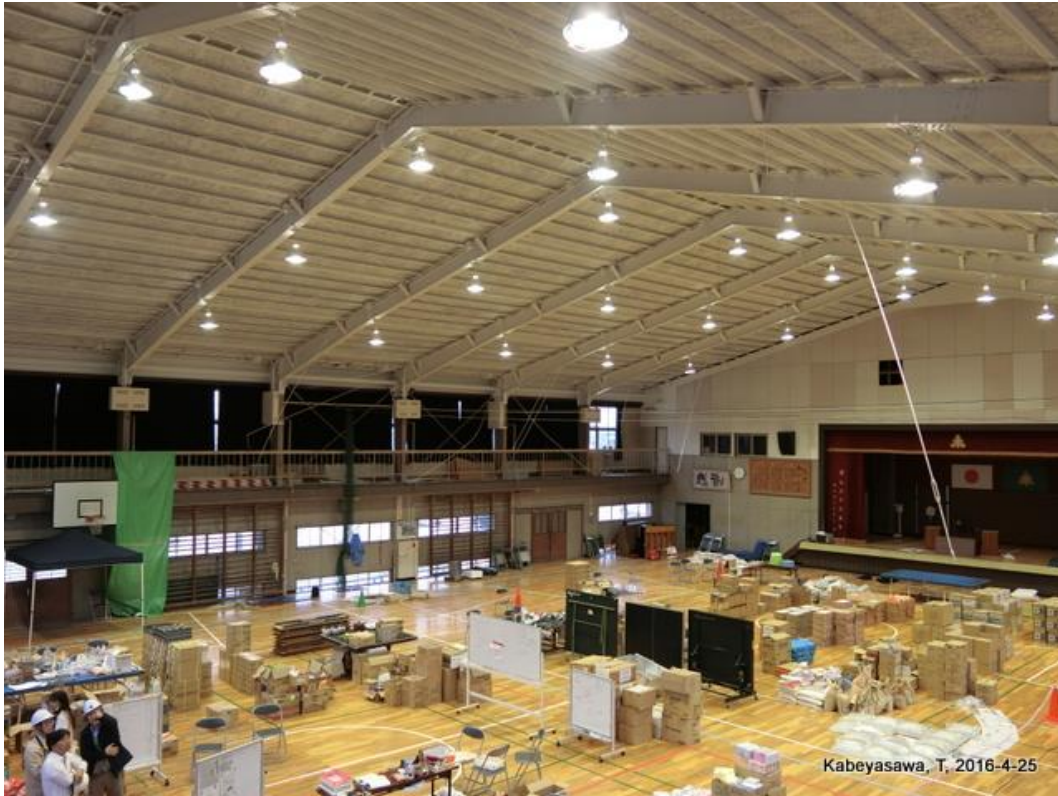
体育館 Gymnasium used for stock spaces under broken and hanging braces
