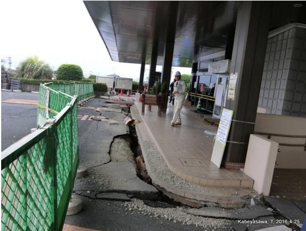
M 役場（周辺地盤の変状） deformation and settlement of surrounding soils,
