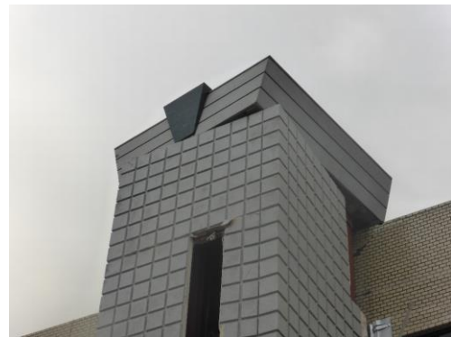
EV 棟の被害 Elevator shaft
