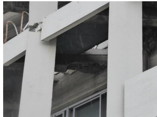
バルコニーを支える斜め梁の損傷 Damage to beam in out frame at balcony end
