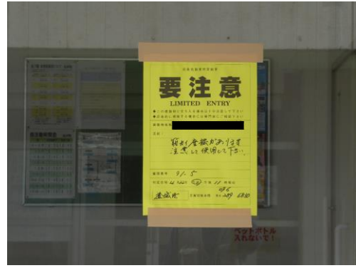
応急危険度判定(体育館) Yellow for main building
