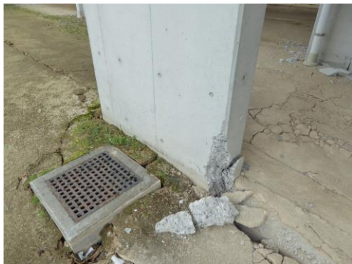
構面外壁の端部筋の損傷 Crushing of wall
