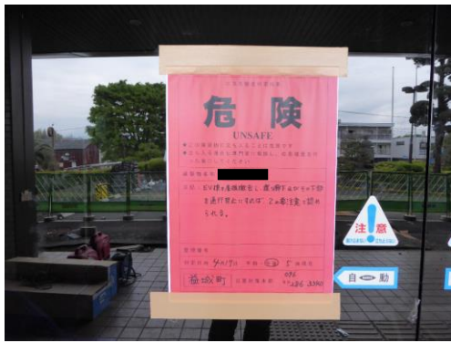
応急危険度判定 Post-earthquake safety evaluation (Red: danger and evacuated)
