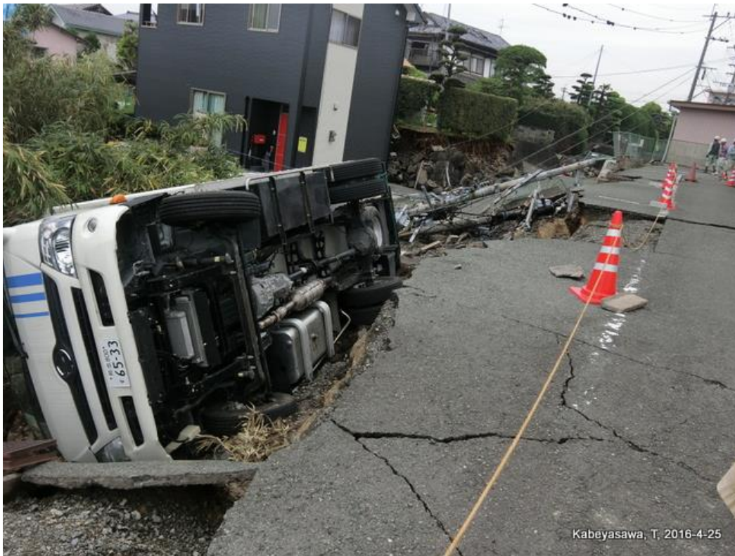
M 役場（周辺地盤の変状） deformation and settlement of surrounding soils,
